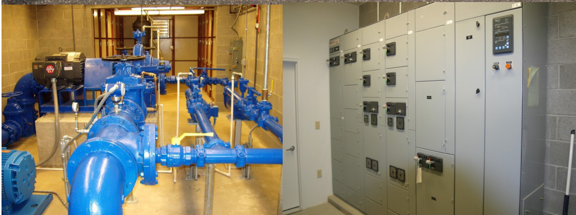
Pumps include a 200hp Vertical Turbine Well Pump; 75hp VFD Medium Flow Pump; (2) 10hp VFD Pumps & 100hp Fire Pump
