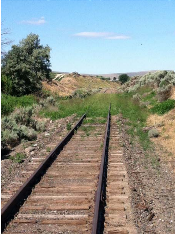
Photograph 5. Vegetation near MP 1992.5
