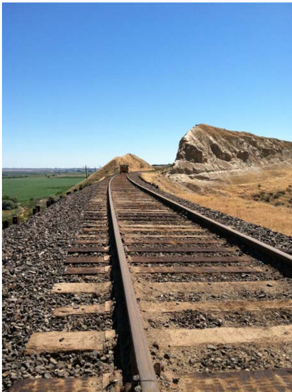
Photograph 3. Ballast Retaining Structure
